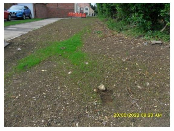
24-level up with topsoil and apply grass seed to take out trip hazard between open space and kerb as necessary across open space pic below.
